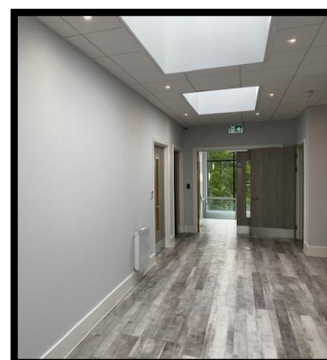
First Floor Landing
