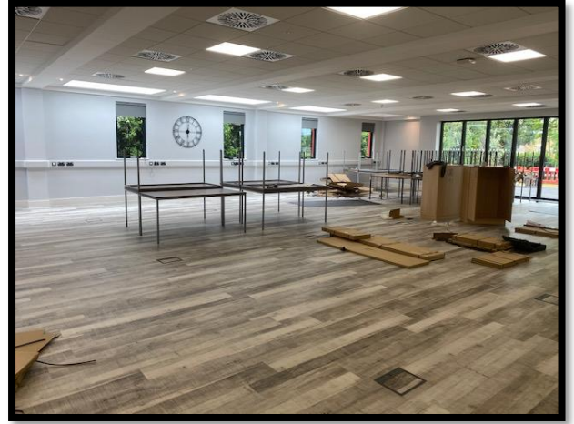
Nearly there on the inside!
